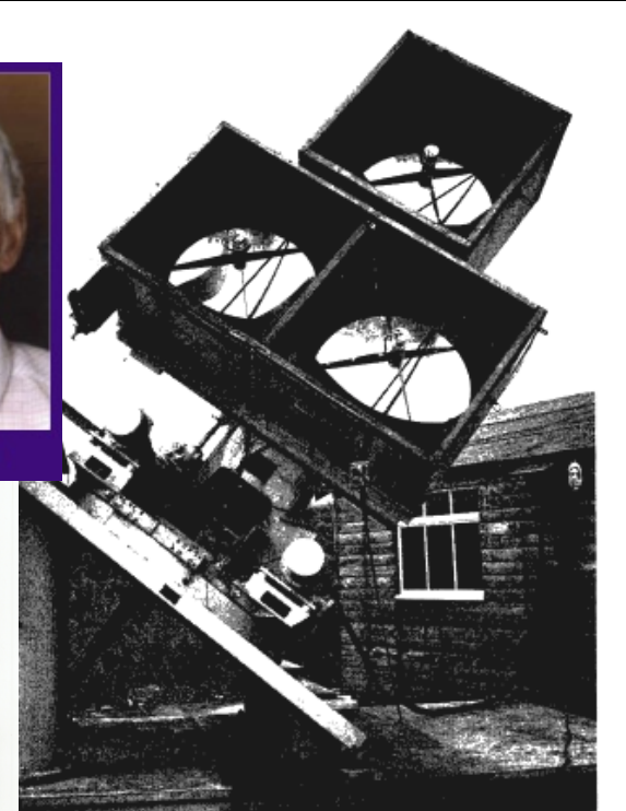
existing light receiver installation at A.E.R.E., Harwell. The bank of three-foot f/0.5 mirrors is mounted equatorially for drift scans.
